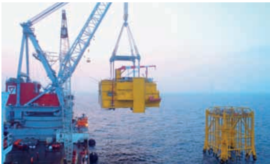
Seaway Heavy Lifting helped complete a wind farm with the installation of a transformer topside.
