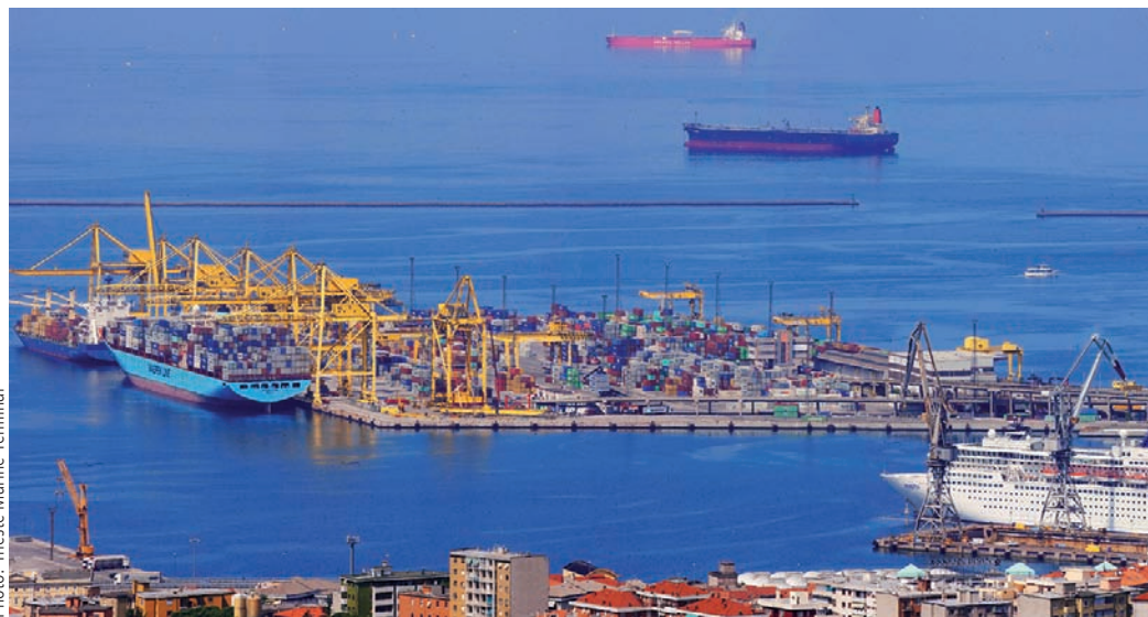
Photo: Trieste Marine Terminal
